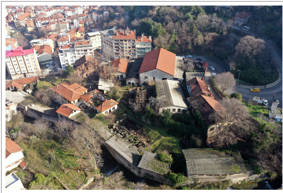
Figure 20. Turgut Yilmazipek silk factory (Bursa) (Osmangazi Municipality, 2025).
